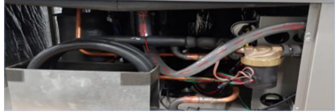
Figure 13: P-trap preinstalled inside the unit
